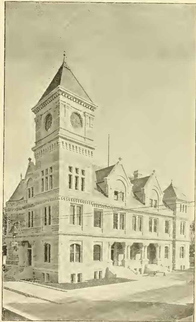
GOVERNMENT BUILDING, MANCHESTER.
